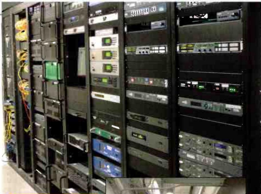
The Technical Operations Center is the heart of Radio One Dallas. The central UPS system, all servers, remote codecs and VistaMax systems can be controlled from here.
