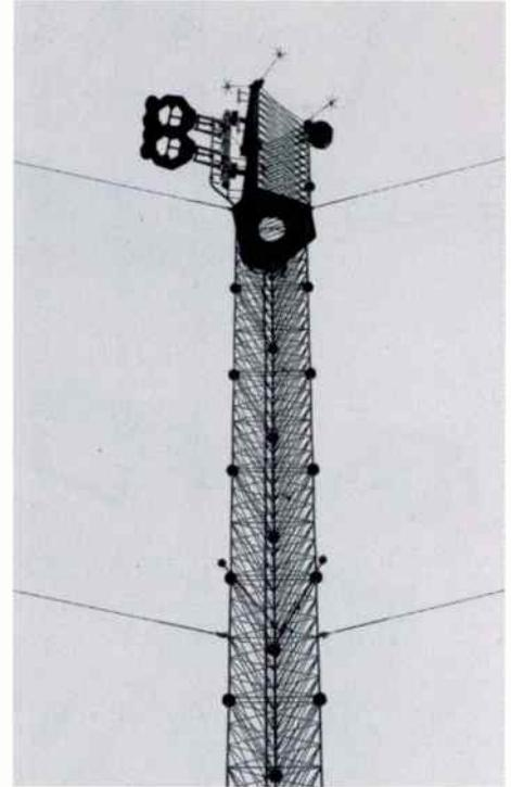
An example of a two-bay nominally non-directional antenna in radomes.
