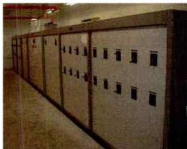
CUSTOM PHASOR INSTALLATION
