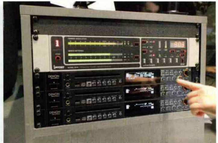
The on-air studio features Denon DN501C CD players and an Inovonics 531N modulation monitor.
