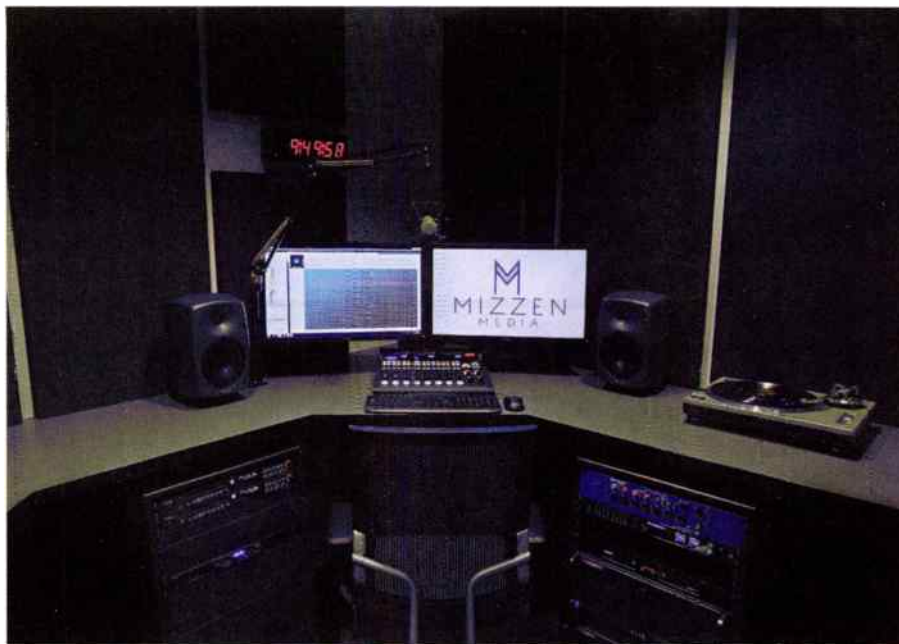
Audio edit bays feature Wheatstone L8 consoles and Genelec 8050B powered monitors.
