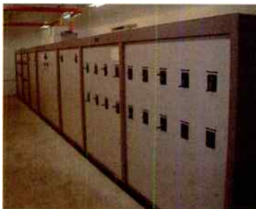
CUSTOM PHASOR INSTALLATION
