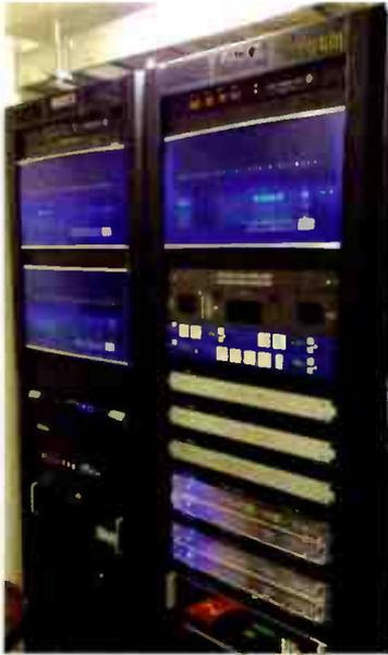
The three-frame 32KD router makes up the heart of the SAS system at Westwood One's Culver City facility.
