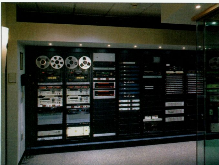
Sufficient rack space and wiring capacities are essential to flexible station operation.
