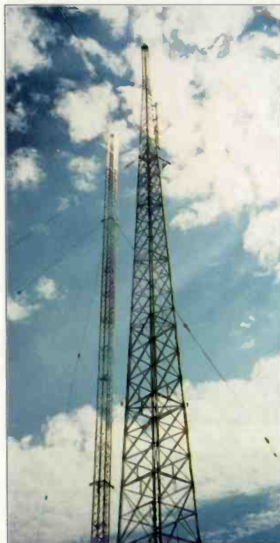
Multiple transmitter facilities can live and work together and save some costs.
