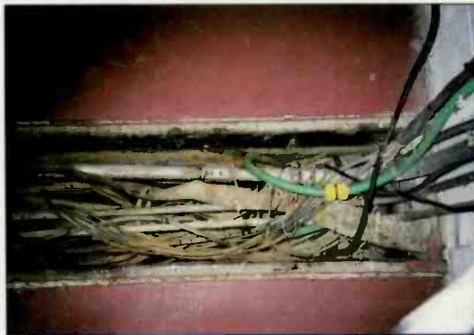
Wiring troughs are fine, but not if you don't keep them dry. This one has seen deep water.
