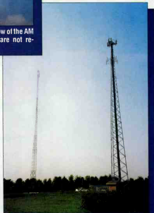
WTRW owns a nine-acre plot which comfortably hosts both towers.
