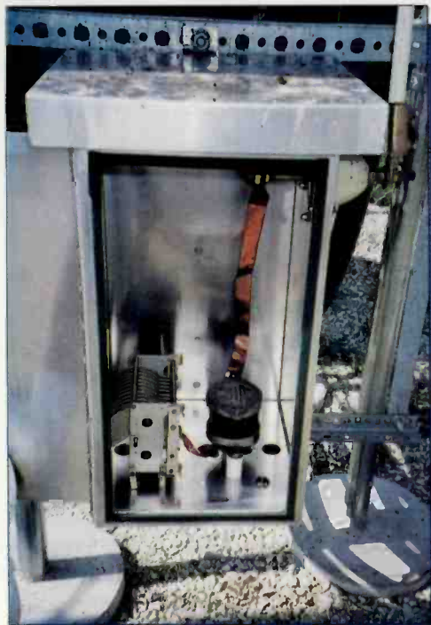
The tuning network on the PCS tower.
