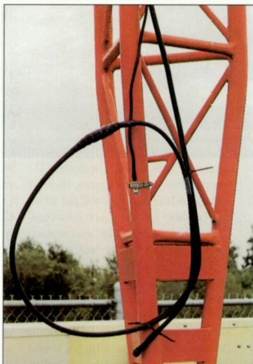
The bond point from the hardline is only held to the tower with a clamp and should be brazed.
