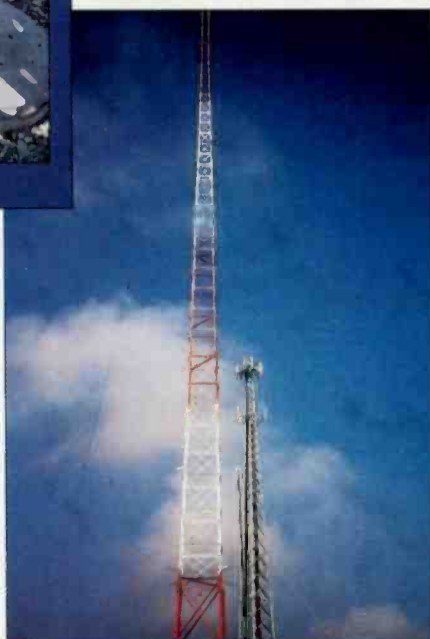
The PCS tower is in the shadow of the AM tower, so paint and lights are not required.
