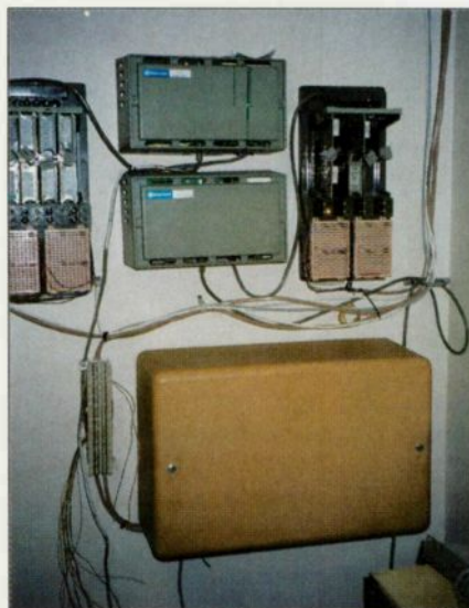
The 1A2 phone system offers reliable call handling, but service and installation can be difficult.
