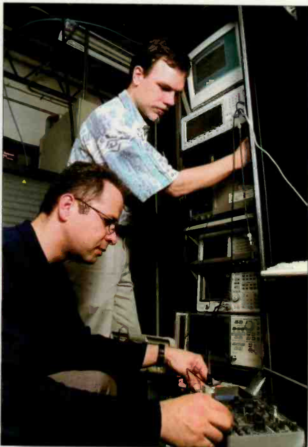
The Lucent tests at WJBK require equipment installation and setup. Greg Nease (standing) and M. Shariat are part of the team putting these tests together.
