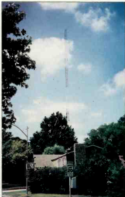
Tower paint condition is only one item in a tower inspection checklist.
