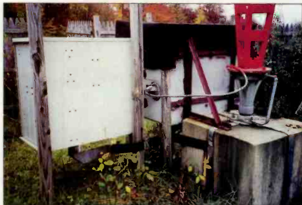
For AM tower bases, check the base insulator, spark gap and all the electrical connections. Photo by Tracey Liston.
