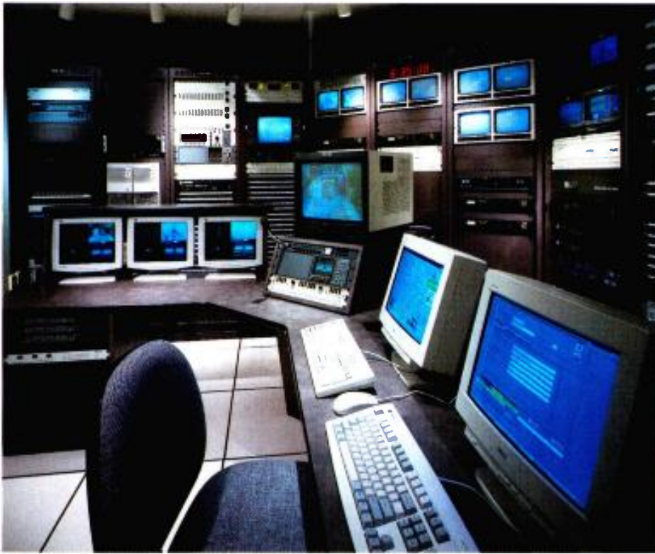
Flat panel LCDs in the Transmission Operations room provide at-a-glance monitoring of network satellite return signals. ILC monitoring and control system are shown at right.
