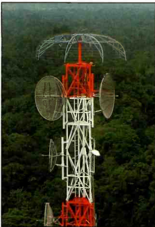
Lightning Eliminators and Consultants' Dissipation Array System, shown above, enables facilities to protect sensitive electronics from lightning strikes by utilizing the natural principle of charge transfer.
