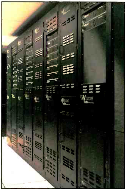
A 512x512 super-wide-bandwidth matrix capable of 4Mb/s through 1.5Gb/s. Photo courtesy Activate. Photo by Richard Bennion.
