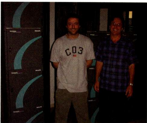
Stefan Sonnenfeld (L), president and managing director of Company 3, with director of engineering Mike Chiado (shown above), utilized Thomson Multimedia Venus Routers to eliminate patch bays in their new facility.
