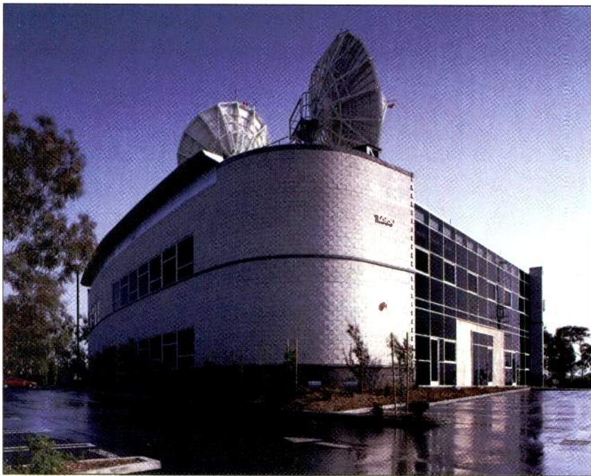
A C-band, five-meter antenna is situated on the roof at Broadcast Services' Los Angeles media center. The antenna is directed toward the Atlantic Ocean region most of the time, facilitating single-hop transmission between Europe and Los Angeles.
