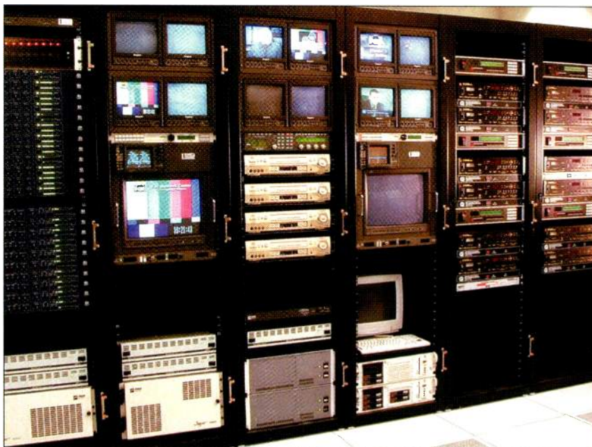
The front-end master-control equipment at the NaviSite.com streaming facility in Andover, MA, includes auto-levelers, phone couplers, audio and video routing systems, and video monitors. Photo courtesy of NaviSite.com.
