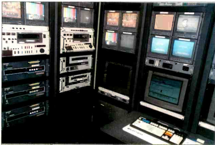
The requirements for the station's new system included file server commercial playback, two-channel operations, automation, modern digital tape format and an SDI-based system. Using a router for primary operations allows stations to rebuild for less.
