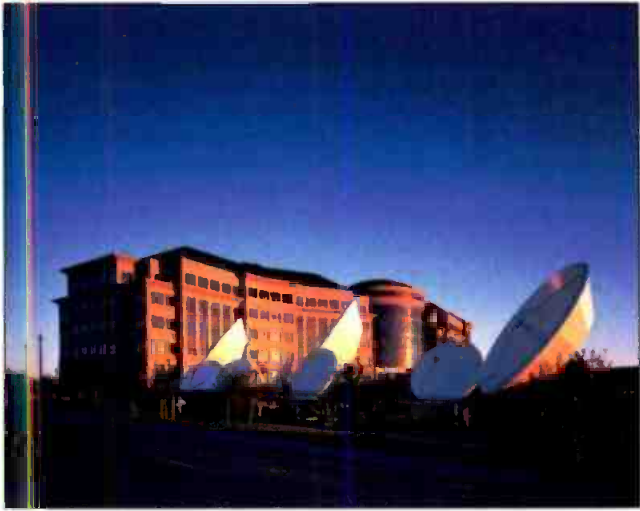
Thirty-six feeds are uplinked from the new facility.
