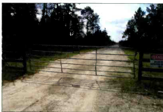
A simple farm-type fence and gate do little more than mark the border of trespass. The warning sign may offer a modicum of deterrence, or it may invite challenge, depending on the reader's frame of mind. Photo courtesy of Richland Towers.
