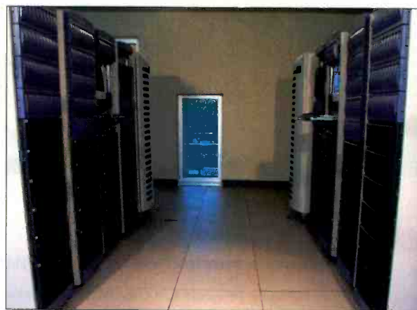
ADIC's StorNext FS manages Turner's broadcast inventory management, the central cache that stores and delivers air material to a network playout server.
