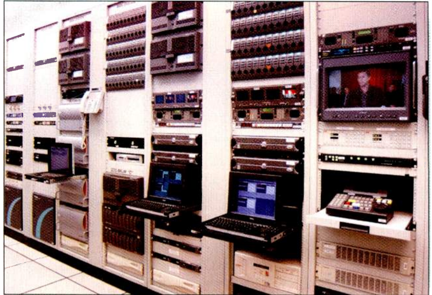
Multiple Grass Valley Open SAN systems from Thomson, consisting of two Profile servers each, hold about four days' worth of content each for four HBO on-air channels. Each movie file is encoded as an MPEG-2 file and stored on hot-swappable Ciprico 146GB drive arrays.
