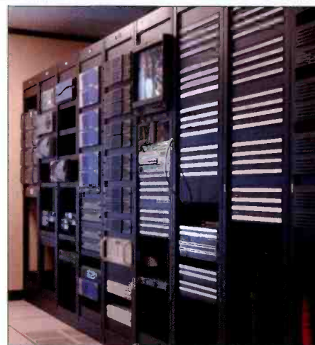
The video row houses equipment for adding graphical elements to network feeds within the air chain.
