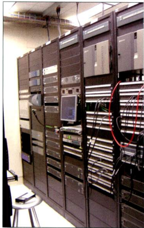
At RAI, signals are managed with Grass Valley Concerto routers, controlled by Encore software, to get signals to the proper destination at the proper time.
