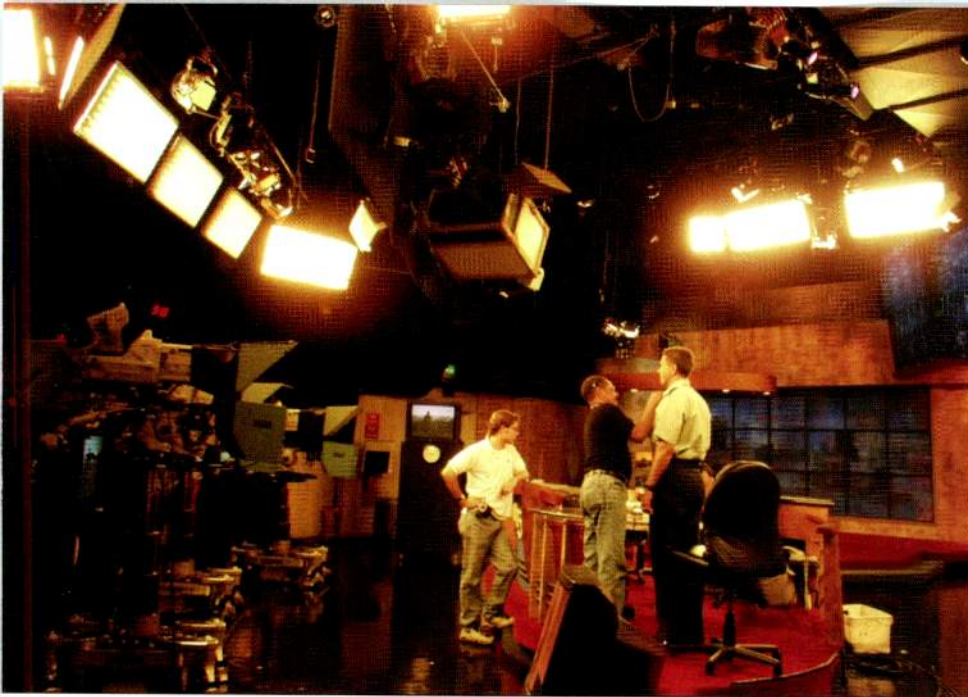
Studios like KTLA Channel 5 News in Los Angeles typically use up 75W/sq ft for lighting compared to 1.5W/sq ft for the average office building. Photo courtesy Kino Flo.
