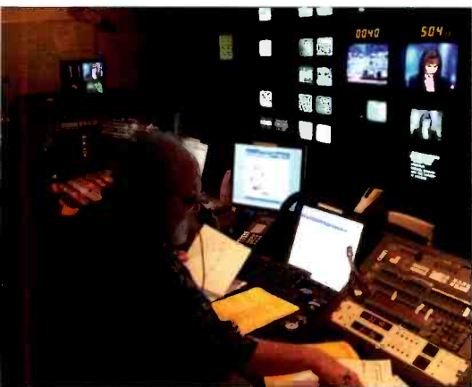
KRON4 streamlined production by integrating BitCentral's Précis play-to-air system with a Canopus Edius nonlinear video editor and Avid iNEWS newsroom computer system.
