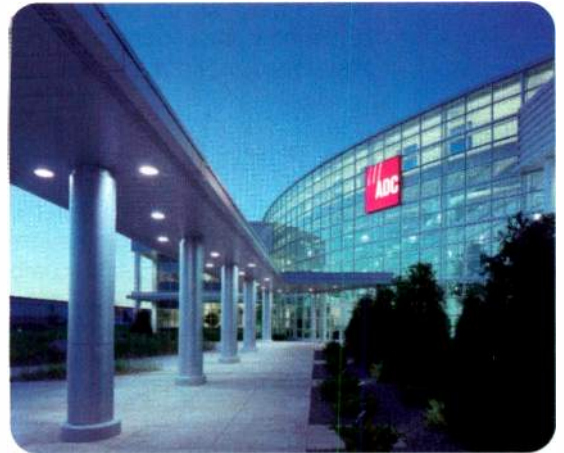
ADC's state-of-the-art facility in Shakopee, MN
