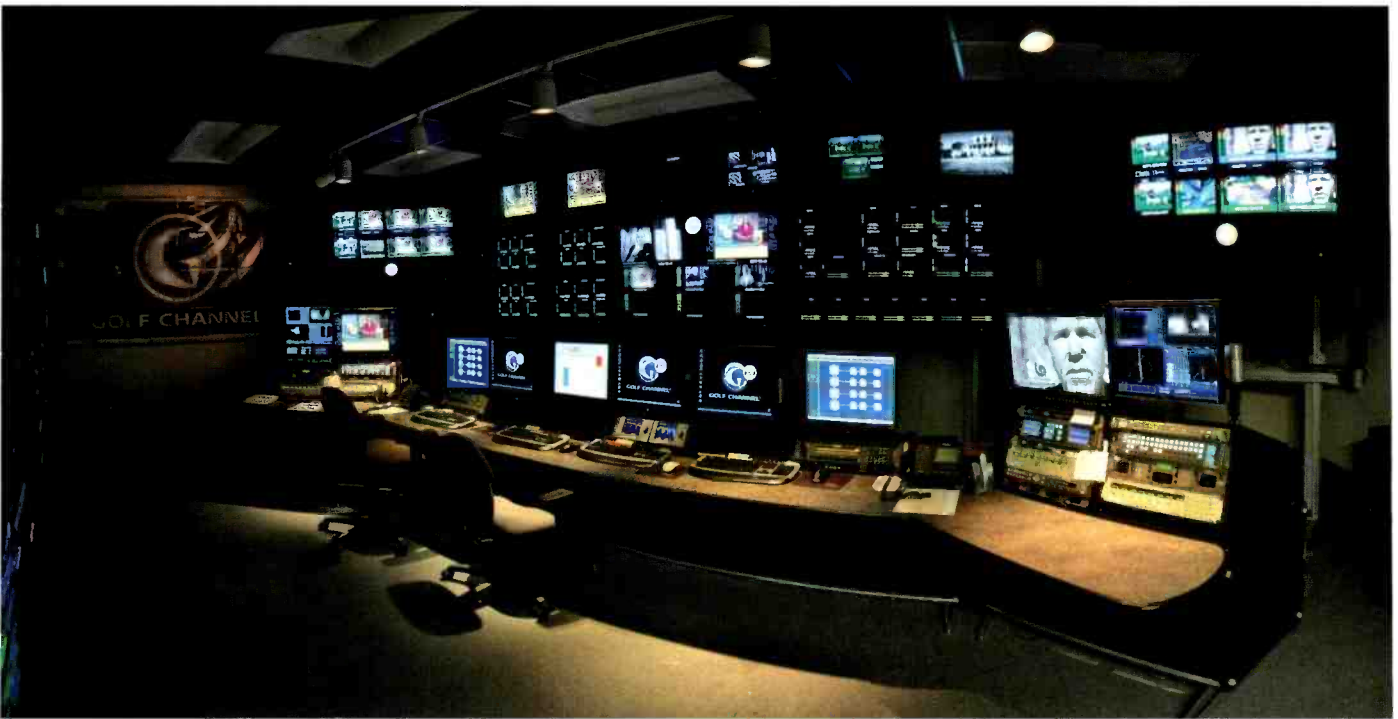
The Golf Channel's transmission operations center maintains and adjusts the integrity of all satellite and fiber feeds, whether inbound or outbound.
