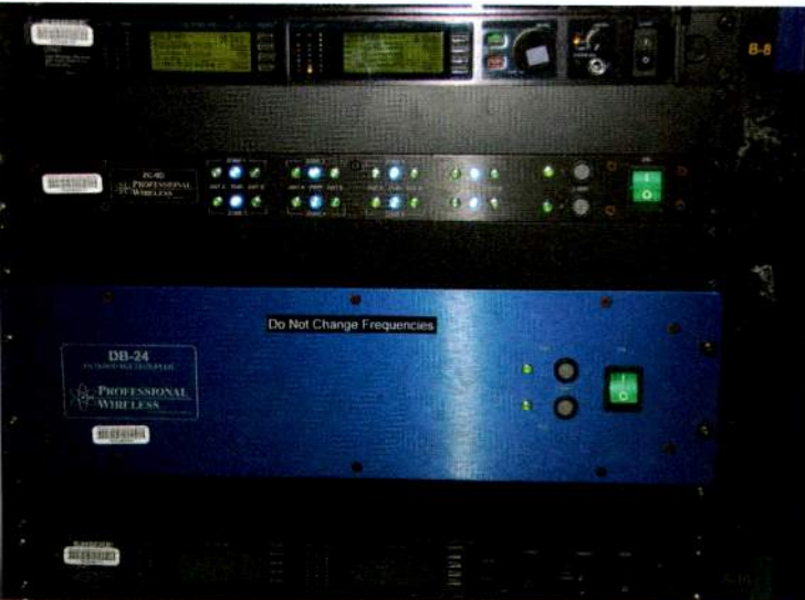
The PWS solution for WMAQ includes a customized 24-output configuration of the company's DB-16 filtered receive multicoupler (left) and a number of off-the-shelf helical antennas (right).
