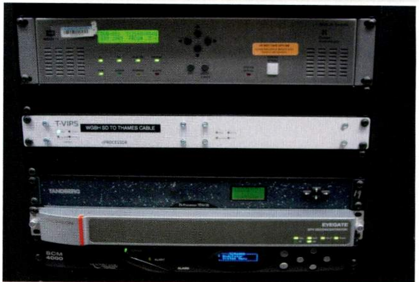
PBS member station WGBH in Boston uses a T-VIPS TVG420 ASI-to-IP video gateway and a CP510 transport stream processor to send its 6Mb/s MPEG-2 SD feed to Thames Valley Communications' headend for wider distribution.
