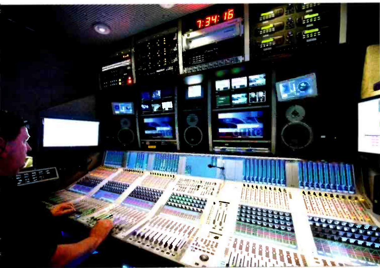
Shown here in the DutchView DV8 OB van, a Studer Vista 9 console is part of the production package built for both low- and high-end productions.
