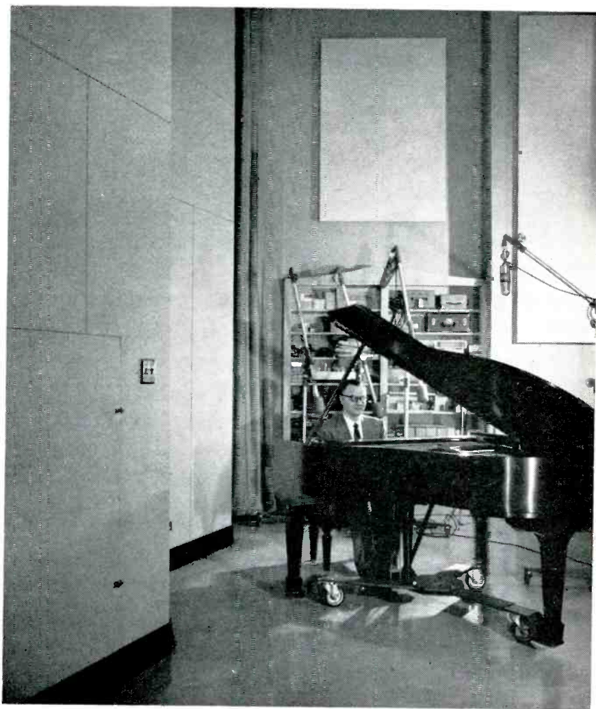
Final pre-recording equipment test in Earl Kennett's newly-designed Carnegie Hall studio. To the left of the piano is a section of sound-reflecting Imperial Transitone movable wall of angular construction. Behind the instrument are sound-absorbing Transite acoustical panels. Covering the floor is quiet-under-foot Terraflex vinyl asbestos tile.
