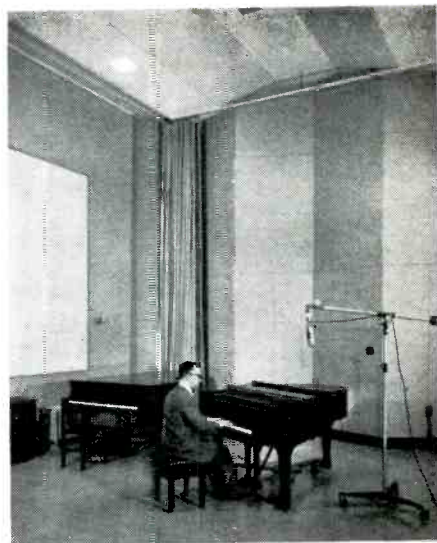
Earl Kennett, an accomplished musician in his own right, plays the piano in a pre-recording equipment test in his Johns-Manville designed Carnegie Hall studio. Facing Earl are saw-tooth-shaped Imperial Transitone movable walls for accurate sound reflection. Next to the piano not in use is an even-finish movable wall, also for sound reflection, and a sound-absorbing perforated Transite acoustical panel. The floor is covered with quiet-under-foot Terraflex vinyl asbestos tile and the ceiling with Permacoustic, a sound-absorbing fissured acoustical tile.
