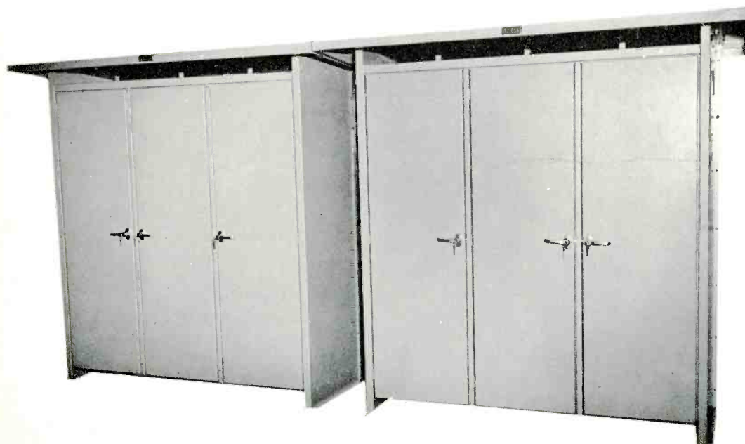
Figure 5. Completed diplexing filters as they will appear at tower base.
