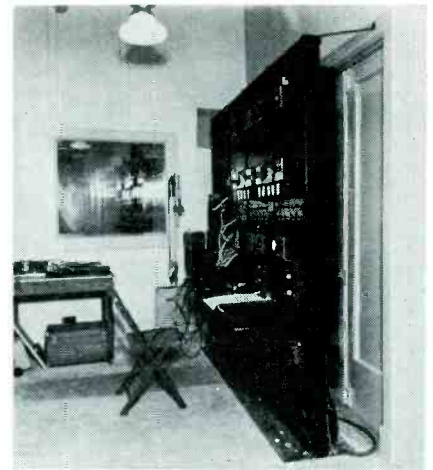
This control-room equipment at WWL in 1922 has almost a modern look.
