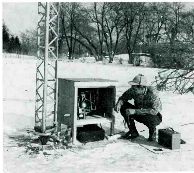
Fig. 2. Tower base and tuning unit at site-test installation.
