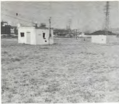
Well-kept transmitter area helps to minimize system - efficiency changes.
