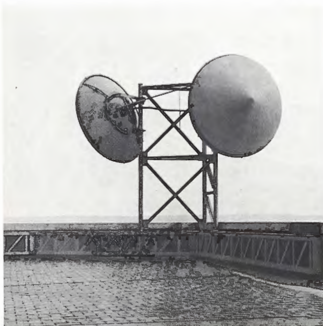
Fig. 2. Passive repeater has heavy steel girder for base.
