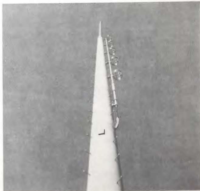
Fig. 1. Views of KCSM tower, antennas. FM antenna is five rings on side of tower; TV antenna forms top of structure.
