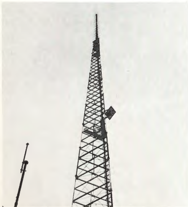
Fig. 4. Passive reflector mounted on transmitting tower.
