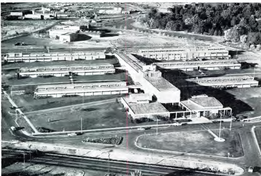
Many activities of ESSA are conducted in this building in Boulder, Colorado.
