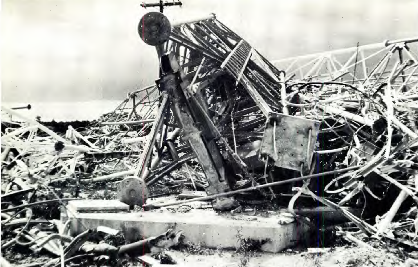
Fig. 1 It couldn't happen in Dallas, Texas, but it did. This is the KDTV tower after a twister hit the transmitter site.
