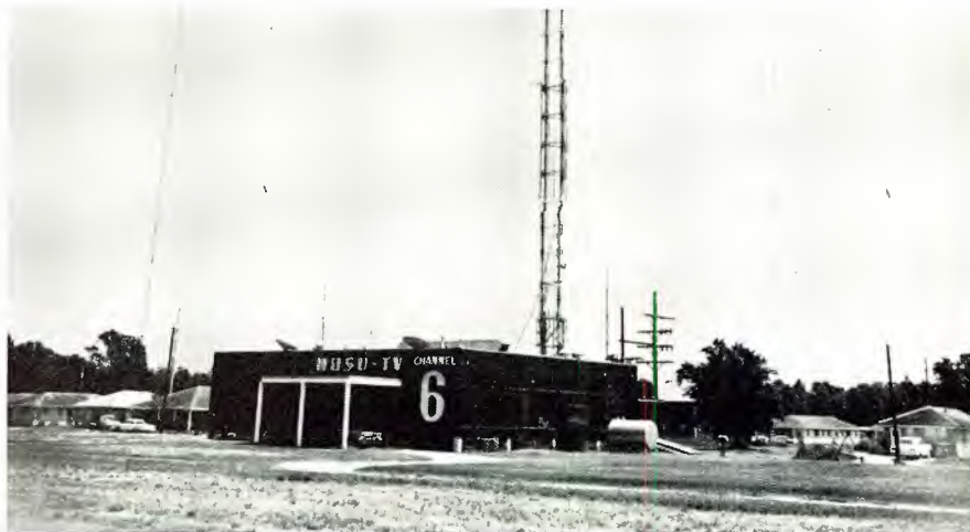
Fig. 2 The WDSU transmitter site showing side location of fuel tank.
