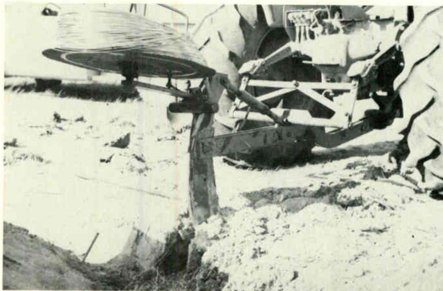
Fig. 2 Home modified farm subsoller used to install the ground system.
