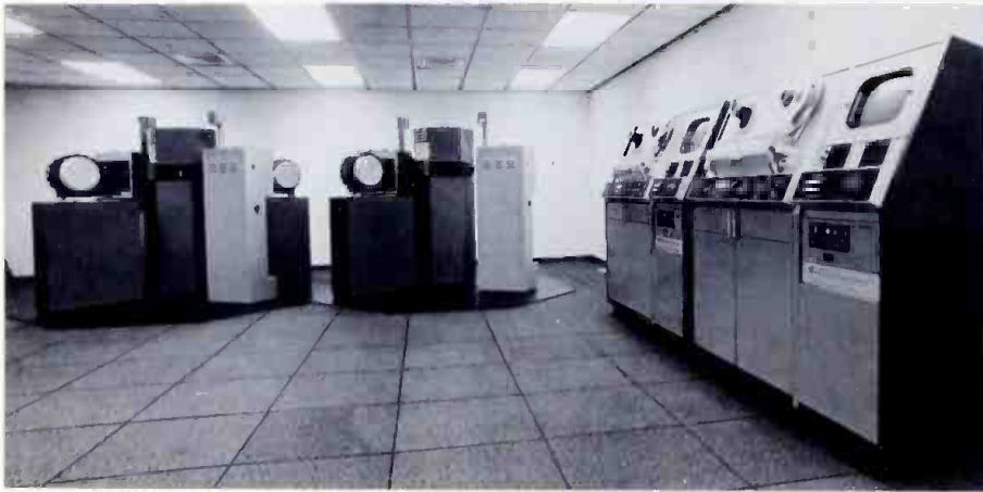
Fig. 2 Film and tape room shown here includes computer flooring and acoustic ceiling.
