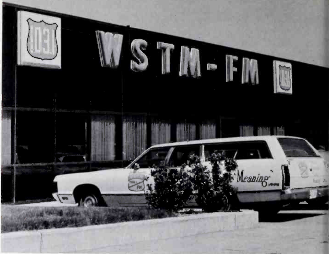
Fig. 1 Front view of the WSTM facility, a special design for FM radio.
