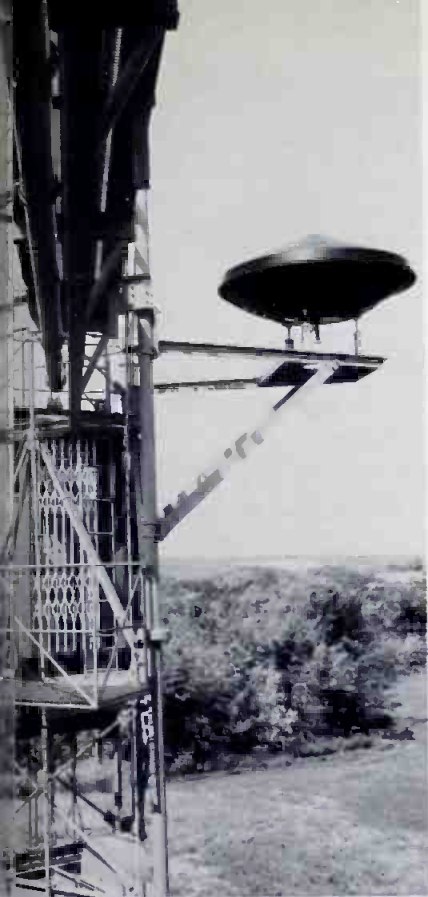
Fig. 3 Note the elevator waiting at the platform. Also, a permanent monorail is shown coming toward the building from just above the tower elevator.
