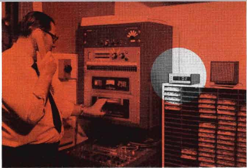
Don McGuire records a telephone "beeper" news report on a cart. At the same time, the electronic timer (right center), interfaced to a recorder, is timing the audio cut. It then holds the readout until the next recording.
