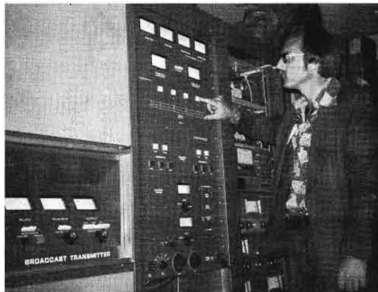
John Davis, consultant to KIQQ, is shown using an RF switch mode controller. The system will put either 25 kW or a 20 kW auxiliary rig on the air.
