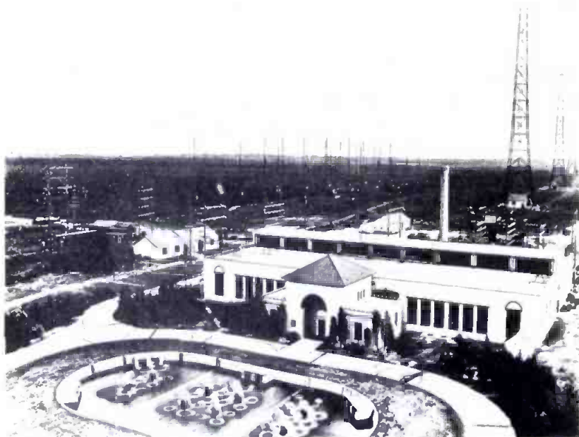
Rocky Point transmitting station opened in 1921. Photo shows 410-foot long-wave towers and the "swimming pool" which was used as a cooling system for vacuum tubes and transmitters. (Courtesy of RCA Corp.)
