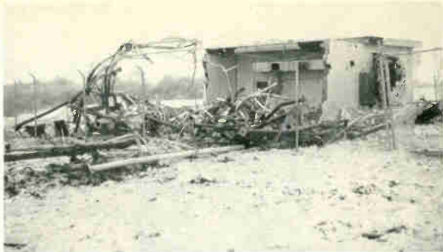
Two-thirds of the Channel 14 transmitter building was completely pulverized by one or more tower sections having fallen on it.
