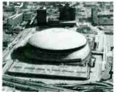
Louisiana Superdome, largest indoor arena in the US, site of WWL's sports broadcast studio shown above.
