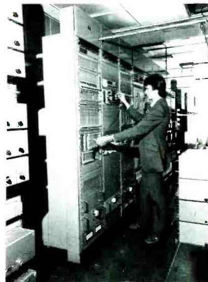
Figure 2 This BBC designed and manufactured 13-channel digital audio multiplex encoding equipment, including a complete reserve set and monitoring facilities, forms part of BBC Radio's distribution network throughout the UK.
