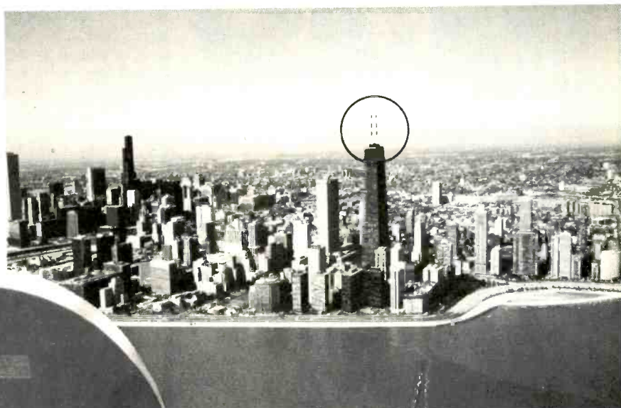
WMAQ-TV DUAL-BAND SUPERQUAD™ RECEIVE SYSTEMS ATOP THE JOHN HANCOCK TOWER, CHICAGO
