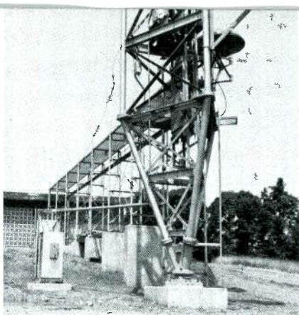
80 ft. horizontal bridge and ice shield.
