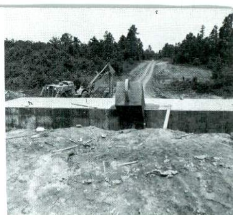
Anchor A-1 capped with 43.8 cubic yards of concrete completing Anchor A-1.
