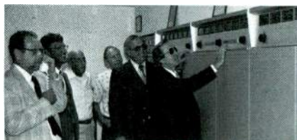
Left to right: Frank Willis, C.E., WFMY-TV; Larry White, Williams Associates (project supervisor); Lee Brady, assistant C.E., WFMY-TV; Jim Key, WFMY-TV transmitter supervisor; R. M. Williams, president, Williams Associates; Ray McMillan, director of engineering, Harte-Hanks Communications, Inc. Ray McMillan turns on TT-50FL.
