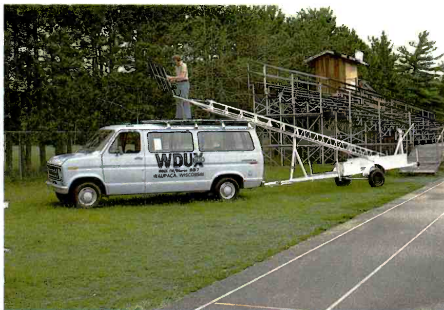
Securing the coax to the antenna.
