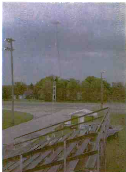
Tower extended to 50-foot height for range of 30-35 air miles.
