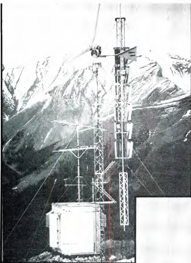
The 50W UHF installation on Pigeon Mountain, powered by the HR2, presents difficult access, even by helicopter.
