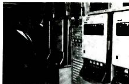
Andy Barry, director, Video Tape Operations, with 1-inch recorders dedicated to adjacent CMX editing room.
