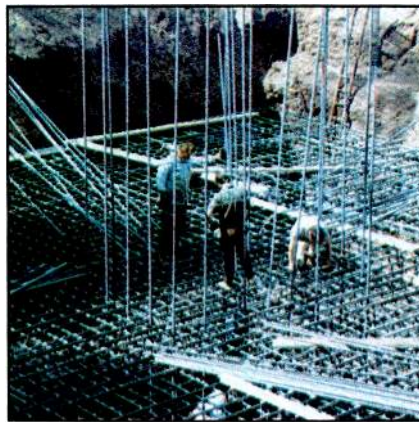
Workmen lay reinforcing steel for footing. Vertical bars will tie into foundation when it is poured. (March 2, 1971)
