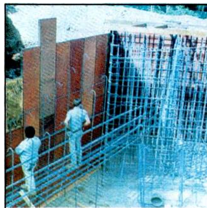
Workmen lay reinforcing steel for footing. Vertical bars will tie into foundation when it is poured. (March 2, 1971)
