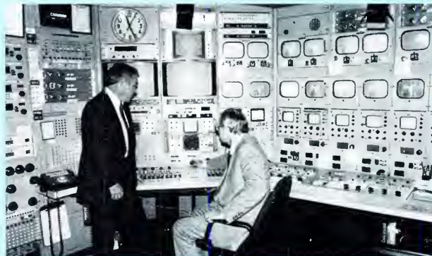
In CBS master control, O'Donnell (left) checks out systems operations.
