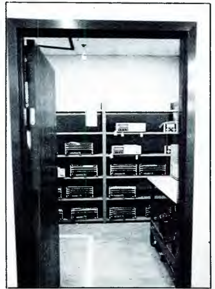
Infant mortality is induced in boards placed in the burn-in room.
