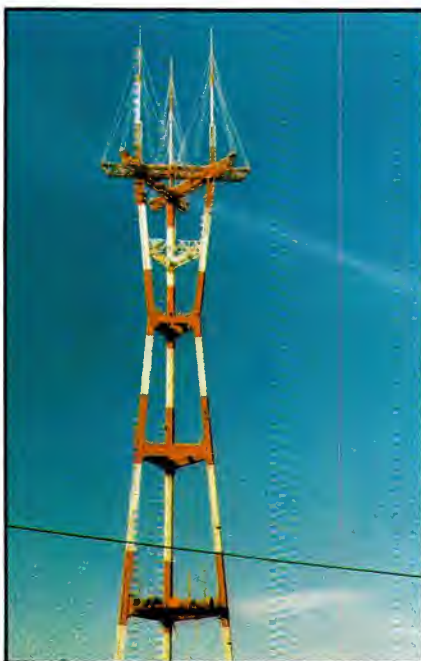
KOIT-FM's transmitting antenna is located on the fifth level of San Francisco's Mount Sutro tower, just below the TV antenna superstructure.
