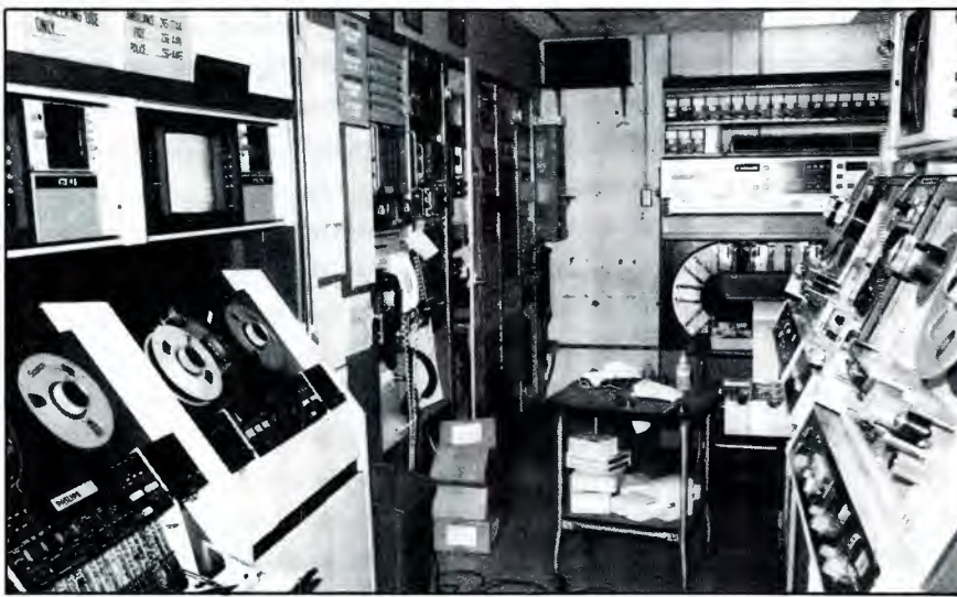
KTHI-TV's tape room houses the station's 1-inch, 2-inch cartridge and cassette tape recording equipment. Machines in this room can be accessed by the master control room or the production control room.
