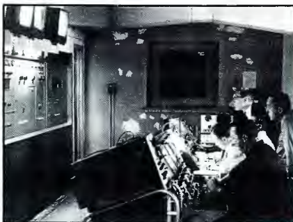
The 1960 WNED-TV master control room, which contained the transmitter and switching equipment, is shown. Note the video monitors mounted above the transmitter.
