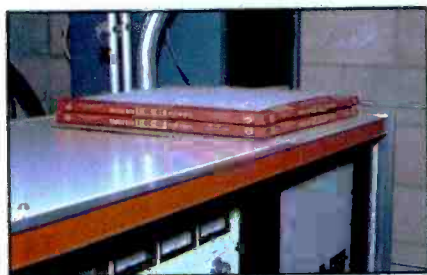
Figure 3. An example of how additional filtering can be added to the air intake port of a transmitter. Standard furnace filter panels can be used and held in position by adhesive tape squares. Alternatively, special computer room filtering material can be cut to size and placed over air intake ports. Care should be taken to ensure that no loss of air pressure inside the equipment results from the additional filters.
