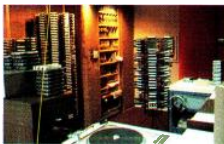
The master control room of WKBW radio in Buffalo, NY. The room shape is an irregular pentagon with extensive acoustic absorption material applied to all surfaces.
