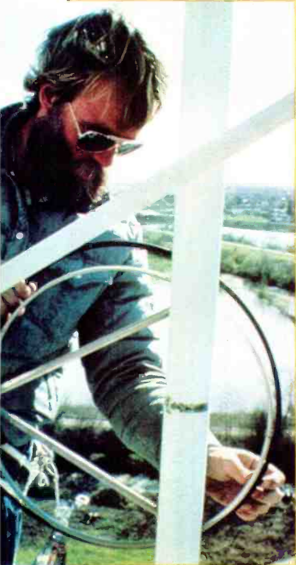
A technician pulls a vertical run of fiber-optic cable on the 1500-foot transmitting tower of KOVR-TV, Sacramento/Stockton, CA.
