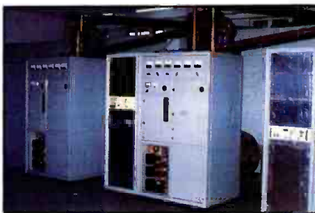
A Chinese-manufactured transmitter at Shanghai TV, which also contains an American-made audio processor.
