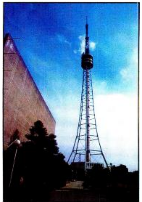
The Shanghai TV tower is 209 meters tall and includes a gondola at the top for observation and equipment placement. The antennas at the top transmit the three local channels.
