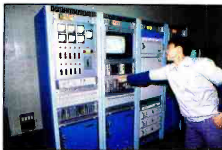
An engineer punches up a studio signal at Shanghai TV. The equipment is a mix of Chinese- and American-built hardware.
