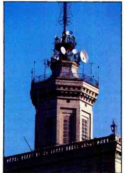
Below, Beijing CCTV is currently housed in a sprawling building that dates back to the 1950s. Both radio and TV services originate there, and are locally transmitted or relayed via microwave to the national network. A new 30-story TV center is under construction. Shown here is the tower above the CCTV building, which serves as the antenna site for the local transmitters.
