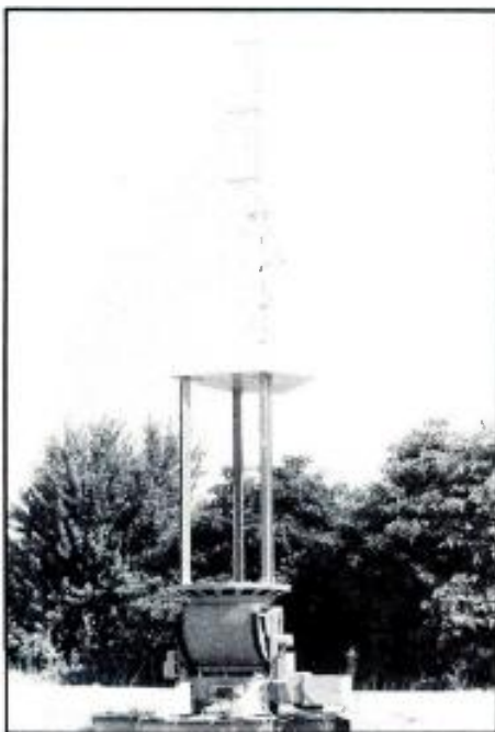
The antenna model in place for measurement. The bottom section of the support is fiber glass. The model tower and pole are mounted above. The climbing cage can be seen on the right side of the tower.
