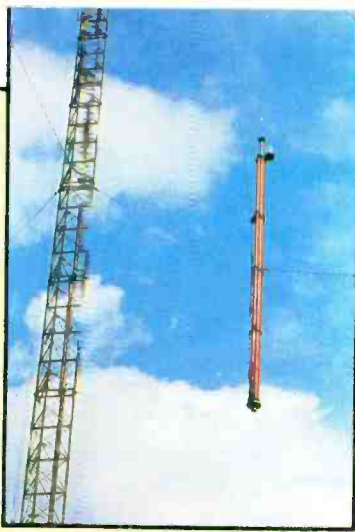
The transmitting antenna being hoisted up the tower.
